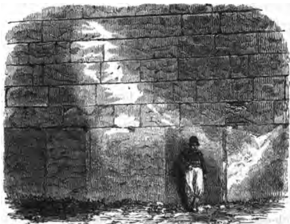
PART OF THE PLATFORM WALL OF THE TEMPLE.
